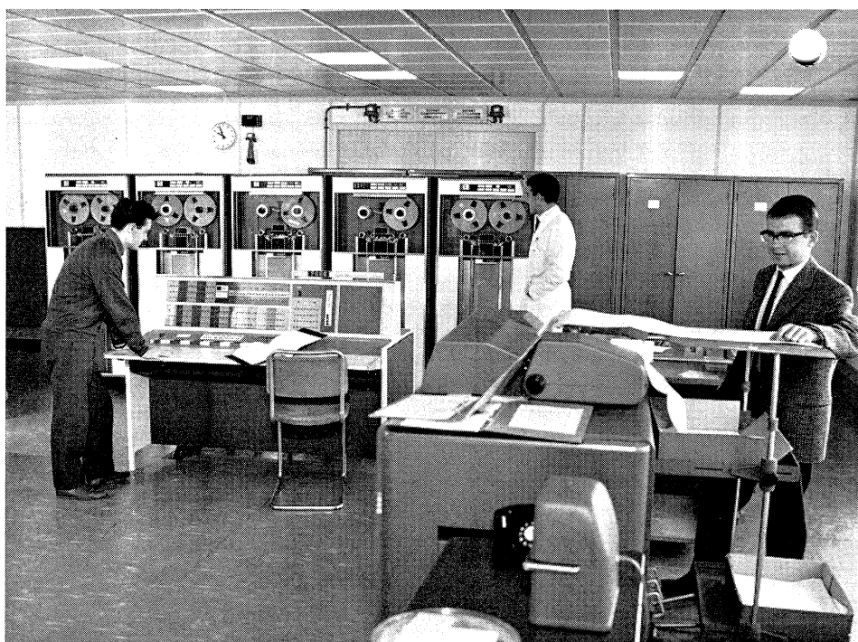
A corner of the IBM 7090 computer room at CERN. At the back are five of the magnetic-tape units, and in front of them the main control desk. In the right foreground is the on-line printer which provides instructions to the operators and information on the progress of the calculations. Also in the picture (left to right) : Richard Milan, Lucio Gourdiolo, and Eric Swoboda.
